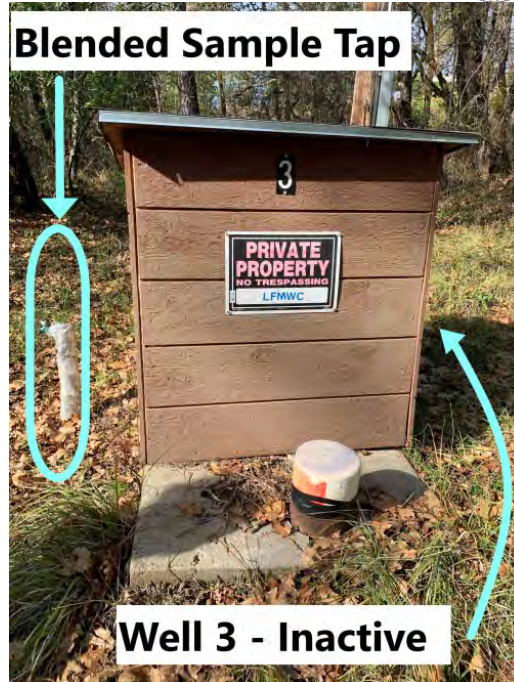
Figure 3: Well 3 Enclosure and Blended Sample Tap
